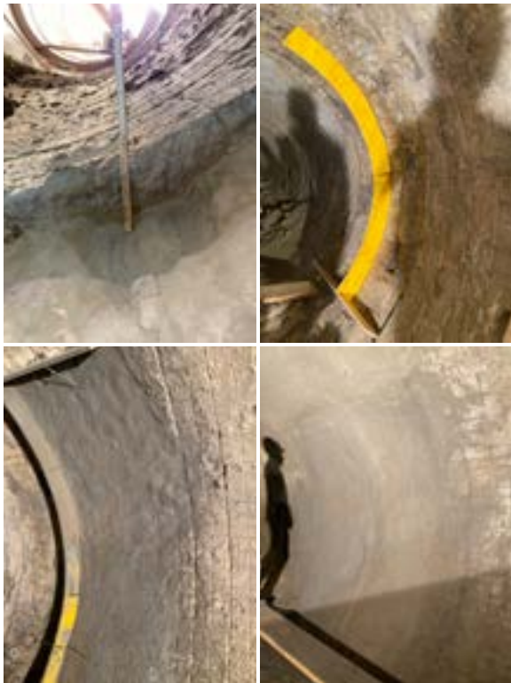
South Austria: Old masonry and discernible thickness of application, field grading, final result after installation.
