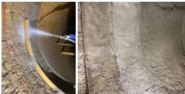
Almost dust-free gunning of REFKO Recovery MG (left) and repair zone after installation (right).
