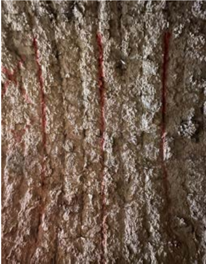
Cleaned surface and marking of the installation fields.
